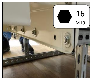
Use housing-collector bolts to securely link to the support stand. Tighten nuts, do not block yet at this point.
